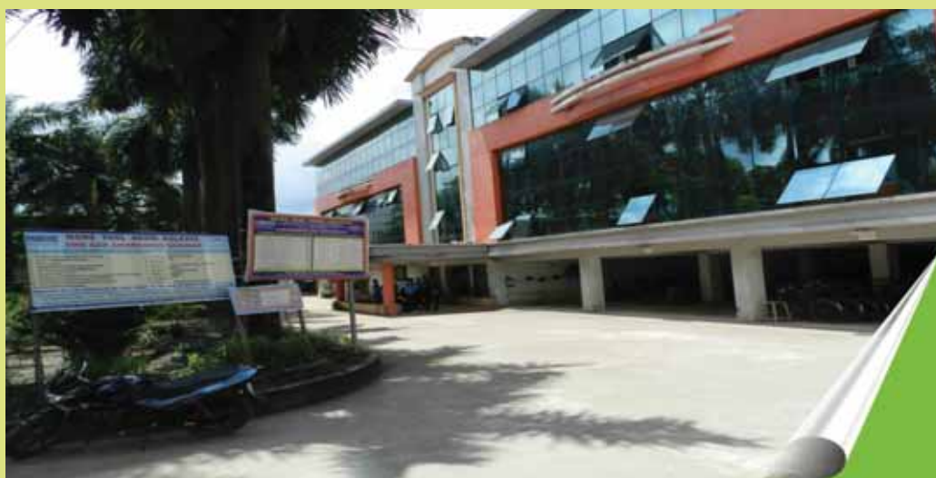
Front View of the Building
